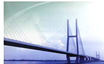
Jingzhou Yangtze river bridge
