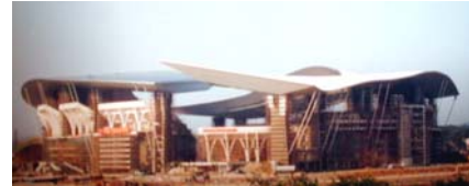
Guangdong Olympic stadium
