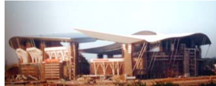
Guangdong Olympic stadium
