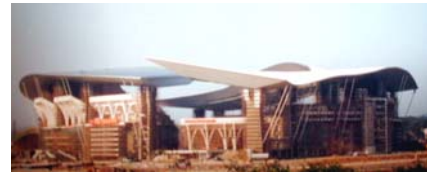
Guangdong Olympic stadium
