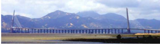
Hong Kong – Shenzhen Western Corridor
