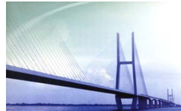
Jingzhou Yangtze river bridge
